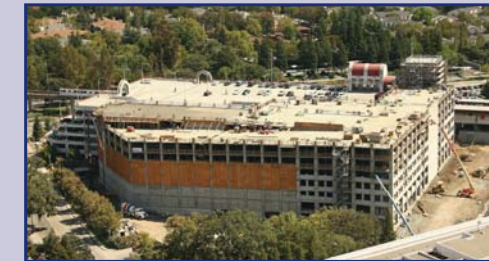
BART Parking Garage
